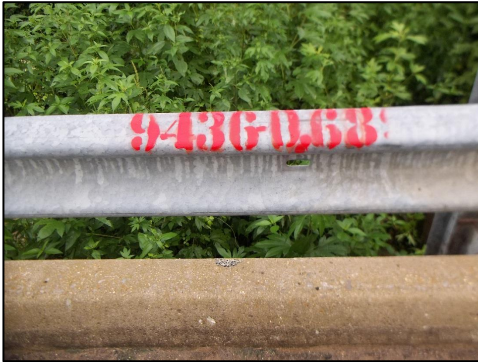
Photo 7: Bridge number on SR-436 Bridge over Reedy Creek
