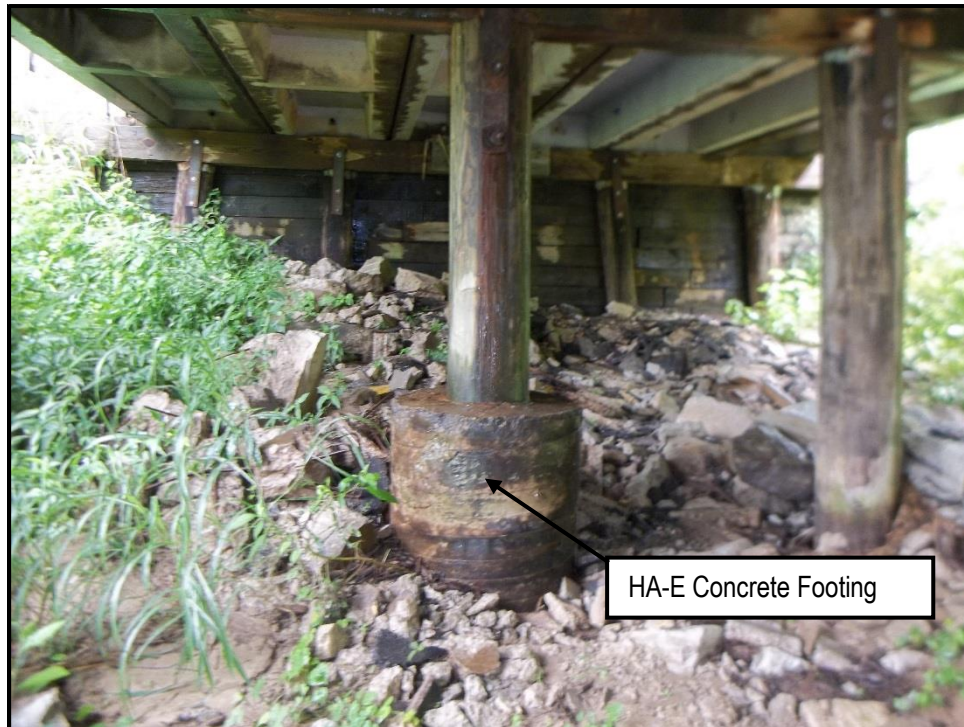
Photo 6: View of HA-E on SR-436 Bridge over Reedy Creek
