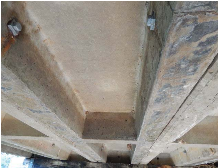
BOTTOM DECK REST OF SPANS
