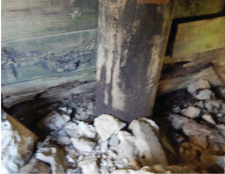
ABUTMENT 2 BREAST WALL
