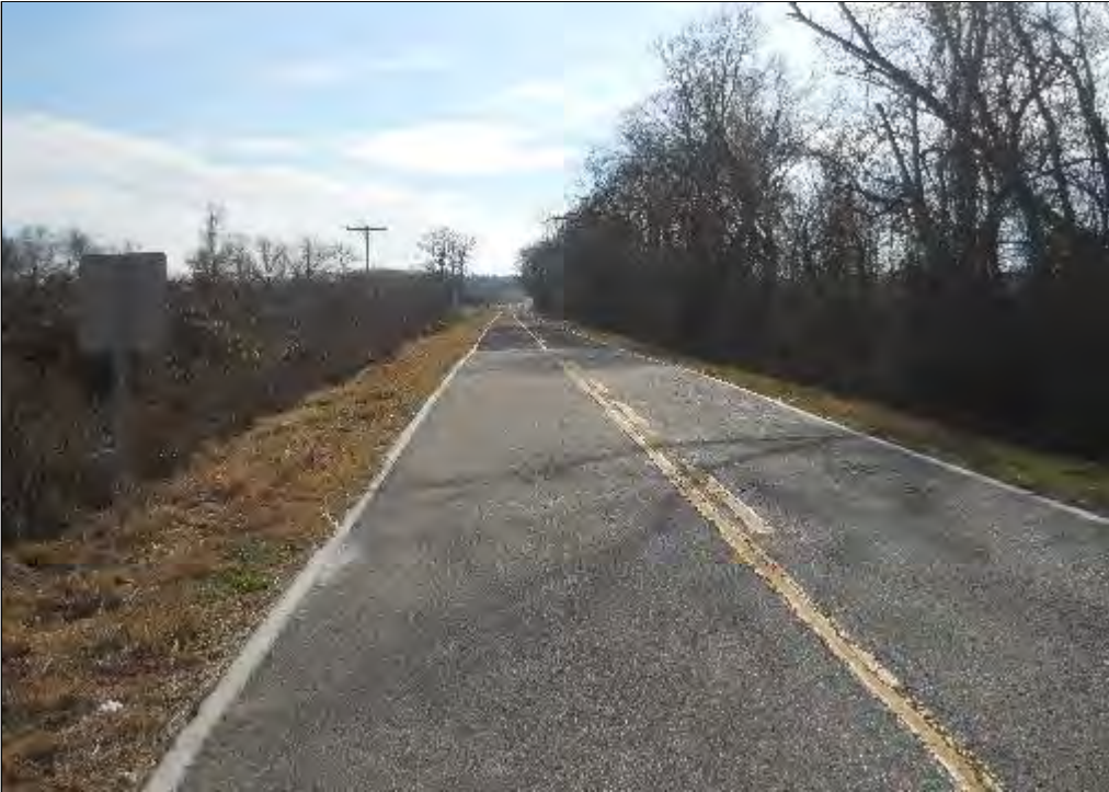
Photo 6: View Looking South From Bridge
