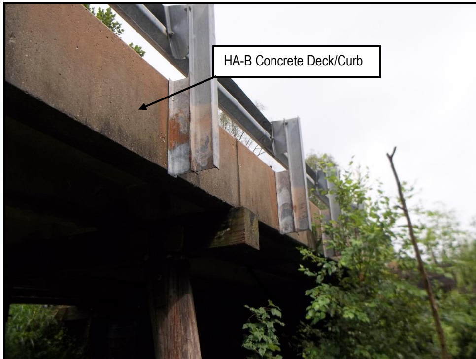
Photo 2: View of HA-B on SR-436 Bridge over Reedy Creek
