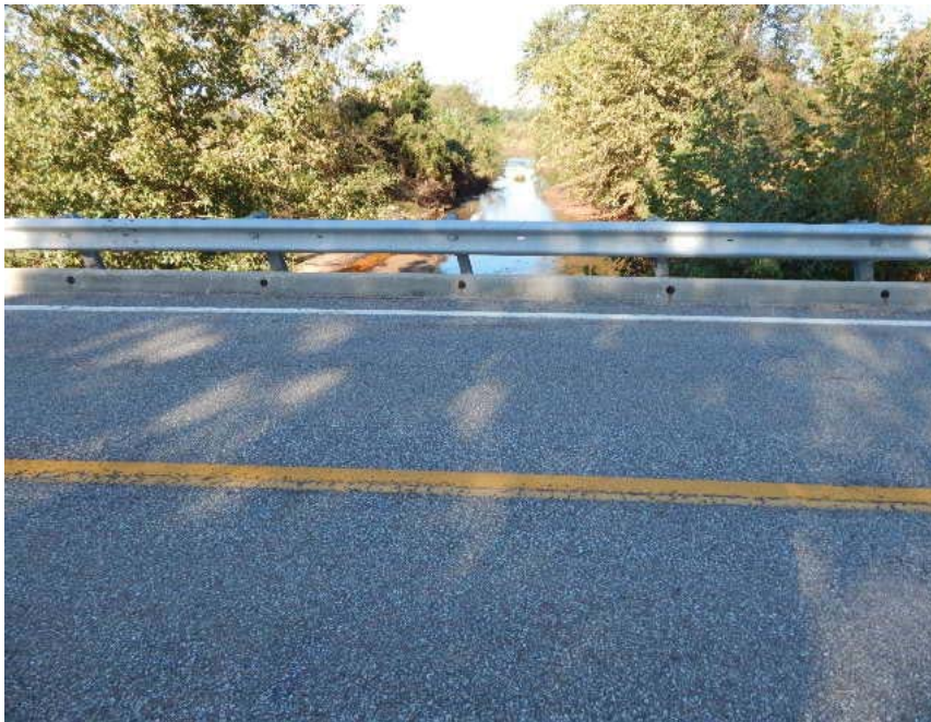
VIEW ACROSS TOP OF DECK
