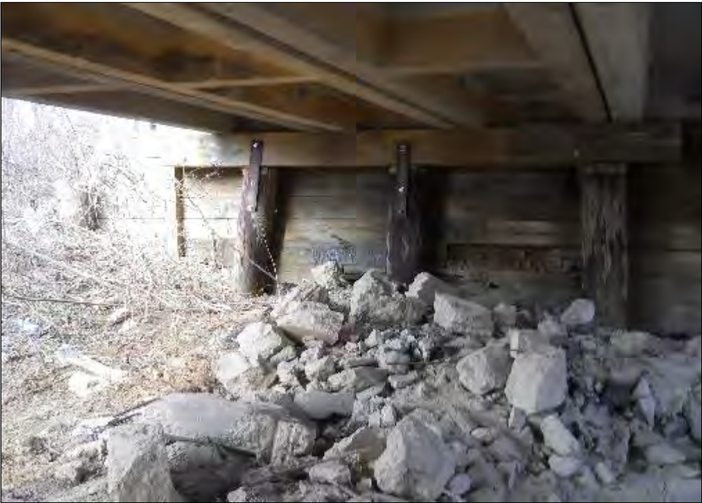
Photo 10: North Abutment Of Bridge
