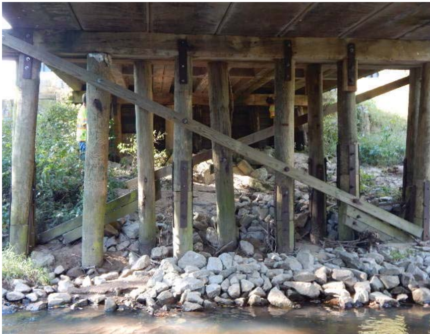
BENT 1 REAR SIDE
