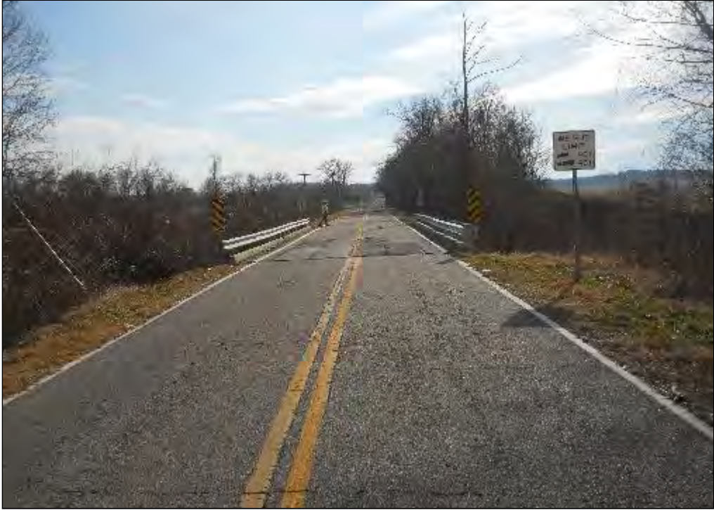
Photo 3: Southbound Bridge Approach
