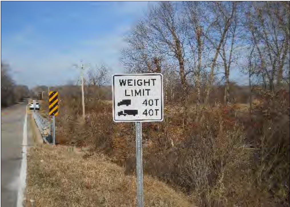
Photo 2: Bridge Load Rating
