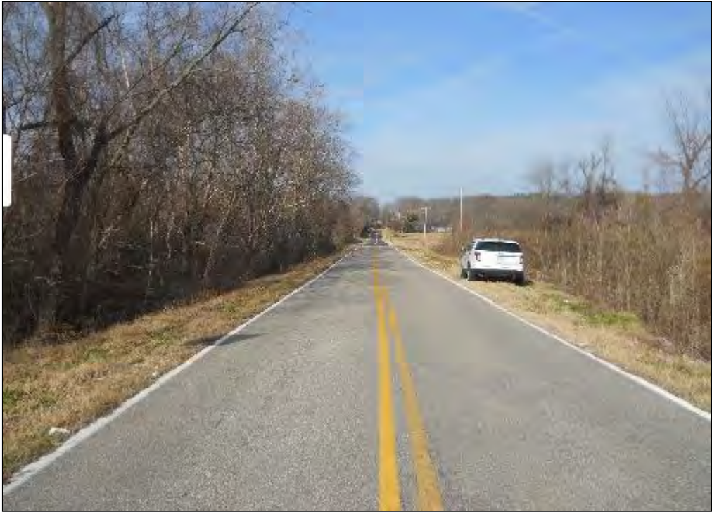
Photo 5: View Looking North From Bridge
