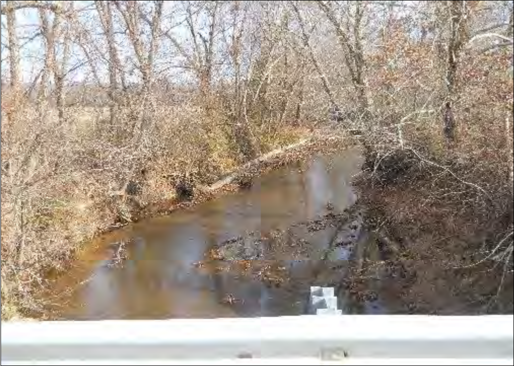
Photo 7: View Looking Upstream
