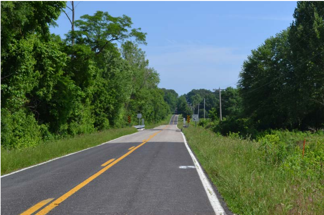
View north along SR-436 toward the bridge.
